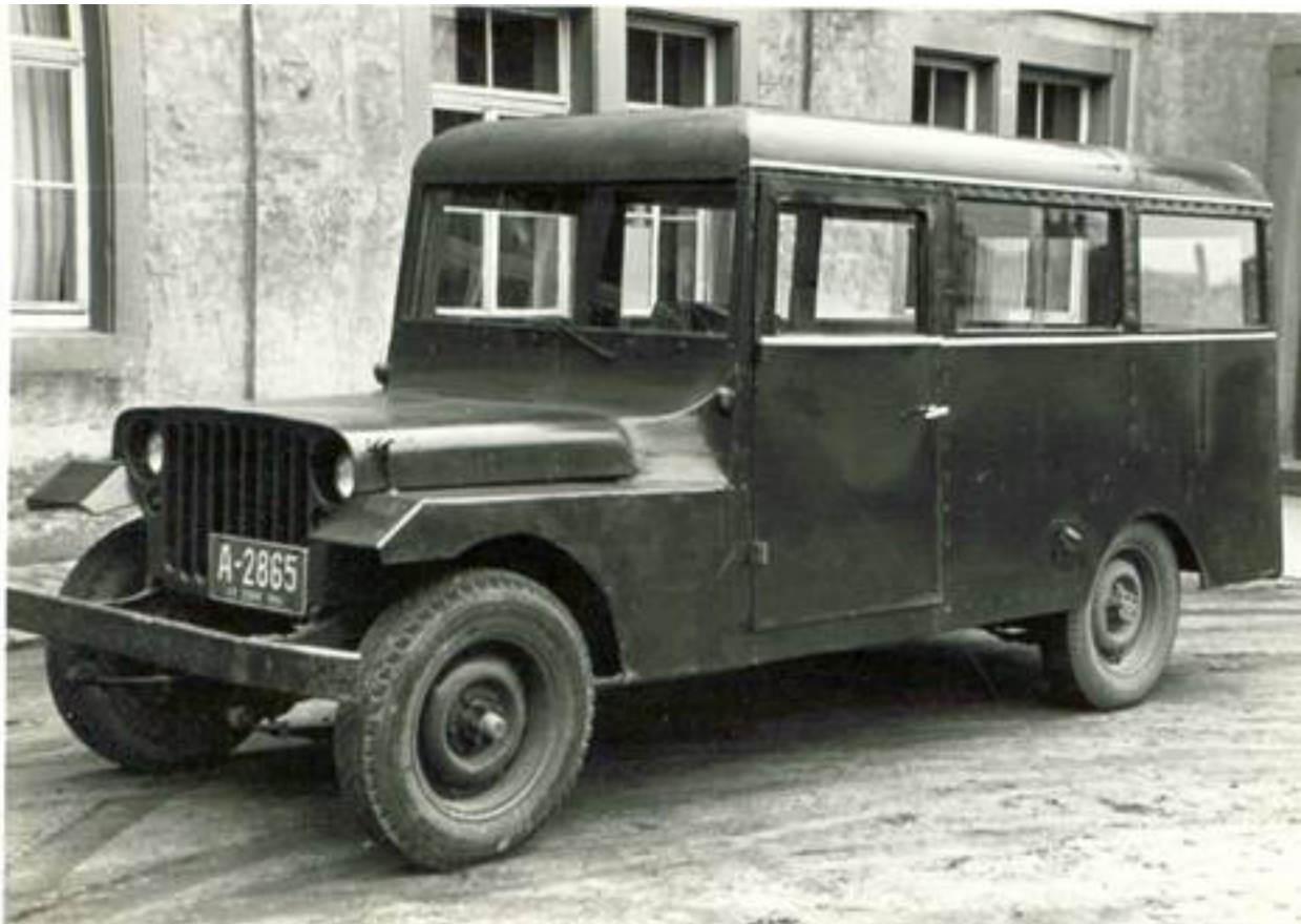
Adam, a station wagon made from a Jeep by MCC workers.
